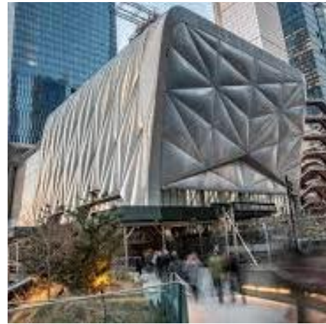
The Shed at Hudson Yards
